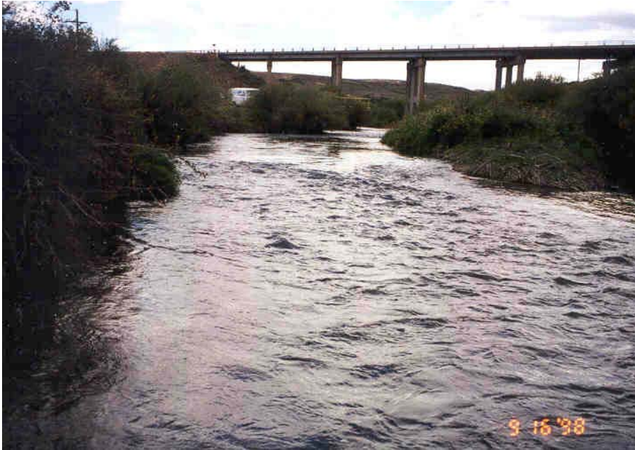
7. Highway 30 Bridge (WBI25), looking upstream on sample riffle.
